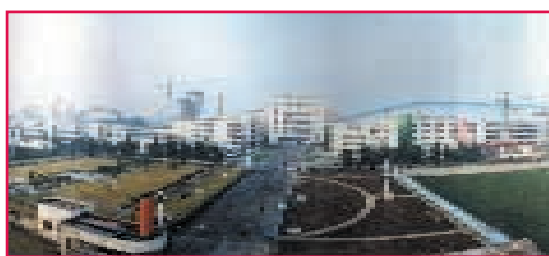
Jining II coal mine
